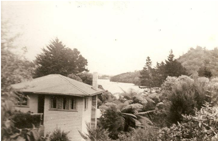
The house at 10 Tui Crescent
