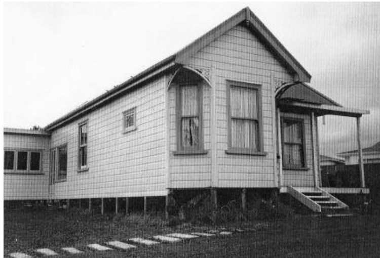
The old Hilder house, after being moved from its original site in 1994
